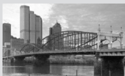
The Smithfield Street Bridge, built in 1883, is the oldest bridge in Pittsburgh and the oldest lenticular truss through bridge in the United States.
