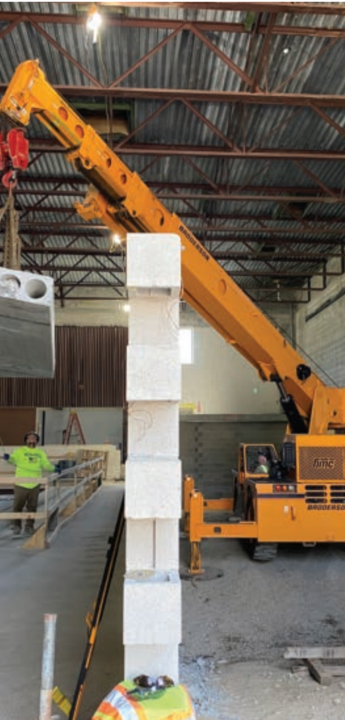
3 The Broderson deploys its outriggers before blind setting the piece, guided by John G. Johnson Construction team members.
