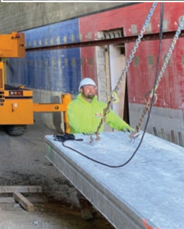
3 The Broderson deploys its outriggers before blind setting the piece, guided by John G. Johnson Construction team members.
