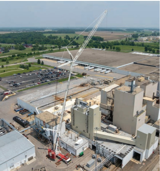
Industrial plant construction in vicinity of Columbus, Ohio. ALL's Liebherr LTM 1350-6.1 with luffer for long-reach, up-and-over picking. June 2025.
