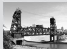
The Norfolk Southern Bridge is historically significant as a noteworthy construction achievement. The bridge's main vertical lift span alone is an impressive and historic structure. It was built in 1957, although some of the approach system is much older than the lift span, and dates to 1906-1917.
