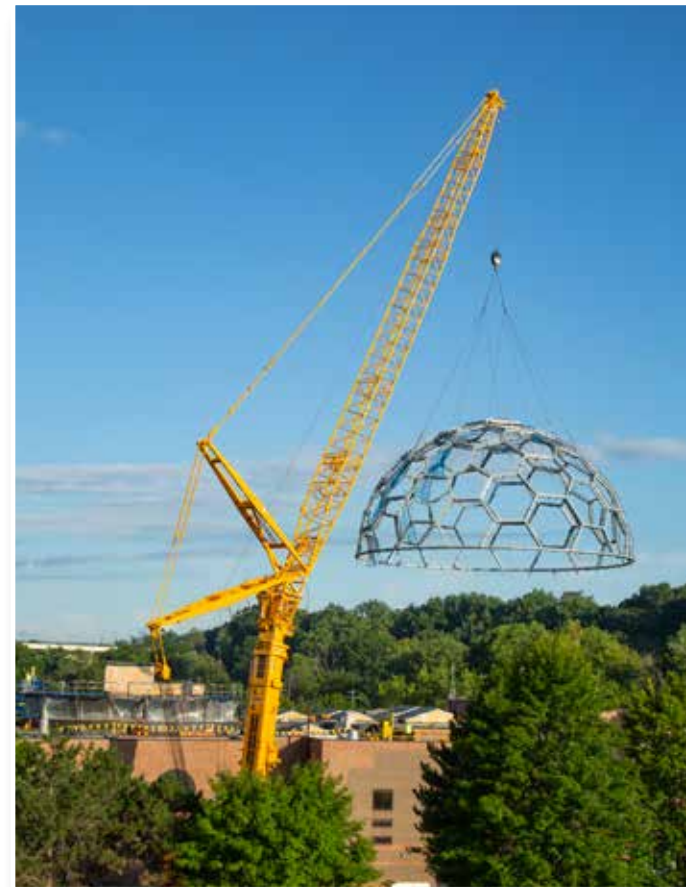
◀ Installation of the new geodesic dome, Cleveland Metroparks Zoo RainForest, Cleveland, Ohio, 2020
