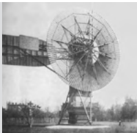
The first known wind turbine in America was designed in 1888 by Charles F. Brush in Cleveland, Ohio. Although large by today’s standards, the machine was only rated at 12 kW and was used either to charge a bank of batteries or to operate up to 100 incandescent light bulbs, three arc lamps, and various motors in Brush’s laboratory.
