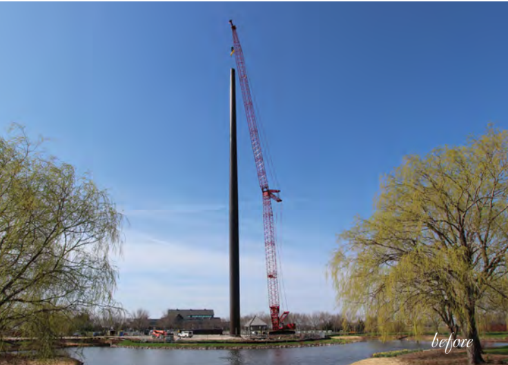
American spirit. Dawes Rigging & Crane Rental, a member of the ALL Family of Companies, builds the tallest flagpole in North America. A wind turbine bears a lot of resemblance to a large flagpole; however, the average wind turbine, at 262.5 feet, is typically not as tall as ACUIITY Insurance's famous 400-foot flagpole. A Manitowoc 16000 Series III (440 ton class EPIC technology crawler crane) was selected for the job.
