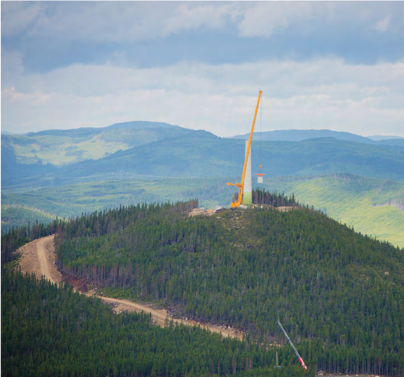
Such great heights. ALL Canada Cranes & Aerials in Mississauga provided seven cranes to help erect 146 wind turbines in phase one of the multi-phase Seigneurie de Beauré Wind Farms project in Beauré, Quebec—the largest Canadian wind power project currently in development. Pictured: ALL's LTM 1500-8.1, with a 258-foot main boom.
