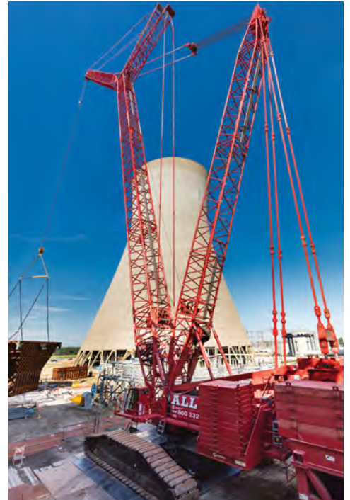
Go big or go home. Our Manitowoc 18000 crawler with MAX-ER (825 USt) lifts massive ductwork for a six-story structure at a natural gas plant in Southern Indiana.
