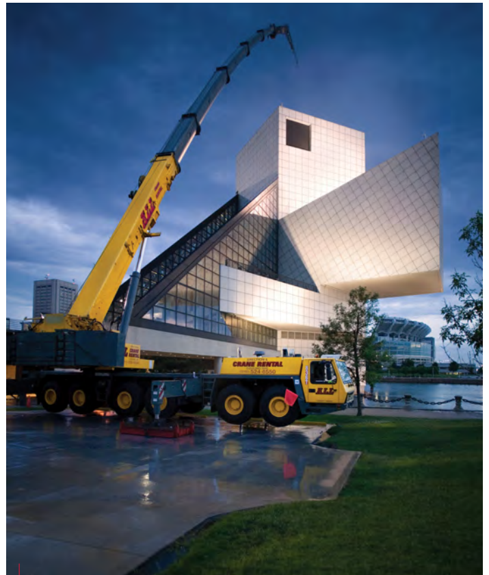
Rock n' boom. In a challenging gig at the Rock & Roll Hall of Fame in 2010, ALL picked an electrical control box for microwave panels off the highest part of the roof. On stage? Grove GMK6250-L.
