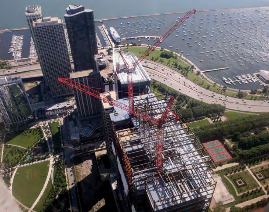
The sky's no limit. The first renovation project in Chicago to build up, not out, the Blue Cross Blue Shield Tower "grew" by 25 stories, building on top of the existing 32 stories with the help of two Potain towers from ALL.
