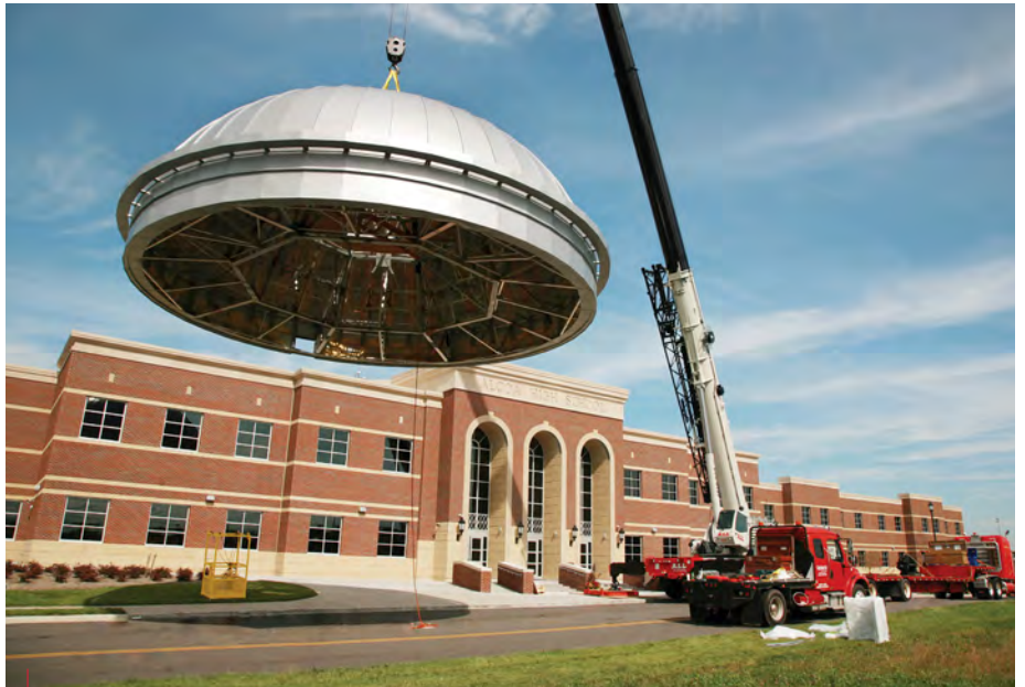
School cap. Alcoa High School in Alcoa, Tenn., received its crown jewel in 2015, a 40,000-pound aluminum dome. ALL Crane Rental of Tennessee provided a 210-USt Link-Belt ATC-3210 to lift and set the dome, its cap, and its spire.
