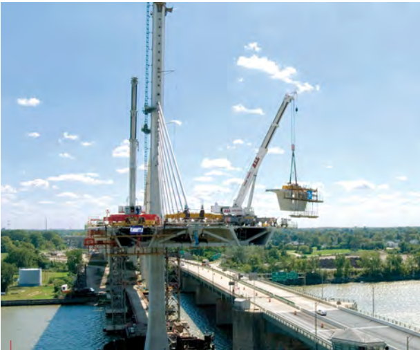
Bridge over "walleye waters." Operators of two 500-UST DeMag AC400 were literally on edge, lifting and placing the enormously heavy concrete segments as the bridge slowly grew 130 feet over the water.
