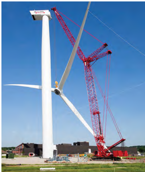
Urban energy. ALL's Manitowoc 16000 builds the $5.9 million, 2.5-megawatt wind turbine in the middle of Cleveland, Ohio.
